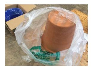
6. We place the filter inside the receptacle, making sure the filter rim is on the 4 foam pieces.
